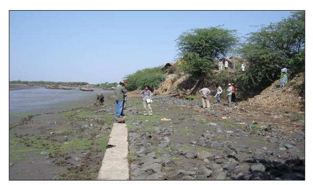
Plate No. 40: Severe erosion and sea wall collapse along northern parts of Narmada estuary, south of Dahej, Bharuch district (Map Sheet no. 46C10NW)
