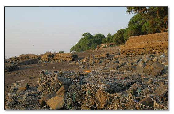
Plate No. 48: Collapse of Sea wall near Umarsadi, south Gujarat (Map Sheet no. 46D14SE)
